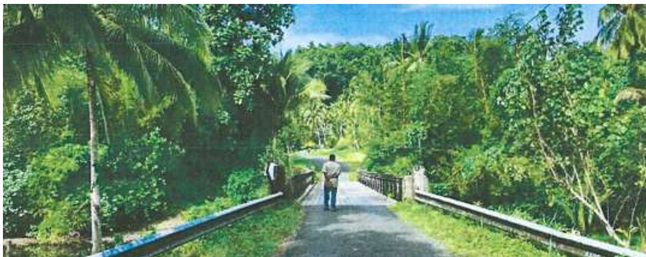
Figure 8: Wutung Bridge, Coastal Highway, Vanimo, West Sepik Province
